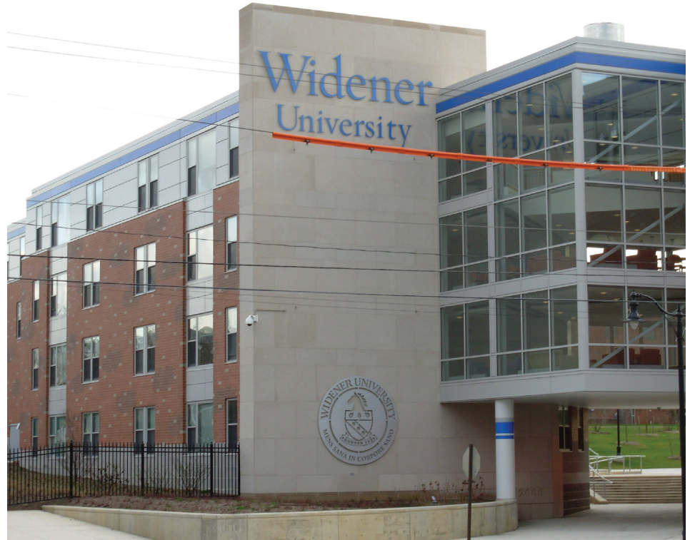
Widener University protected by the IntelliKnight 5820XL panel.
